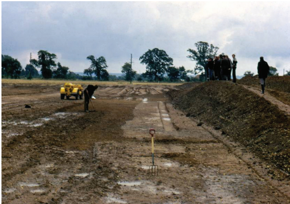
Fig. 6. Construction work on the M40 motorway extension through east Oxfordshire in 1972. Photos: Trevor Rowley.
